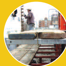
Outriggers that increase the width of working area
